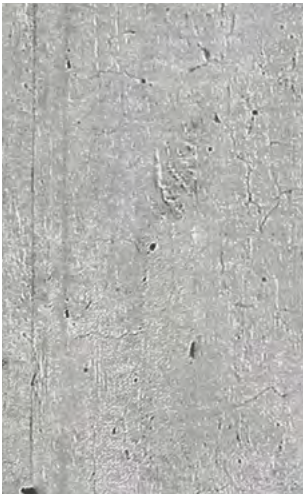
Natural Concrete F2204
